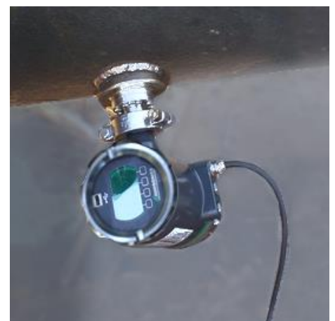
Figure 3: Example of a Weldolet installation
